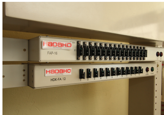
Picture show 12 & 16 fuse alarm panel attach at top DSX Frame
